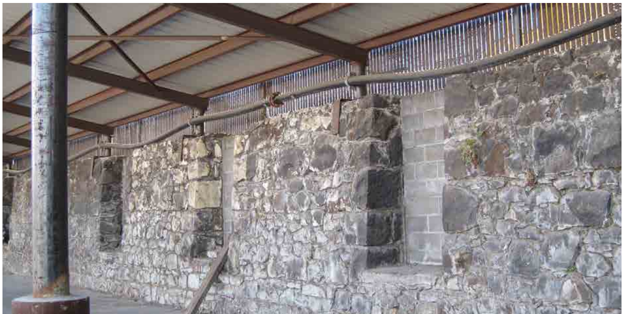
Woolen Mill basalt stone foundation walls
