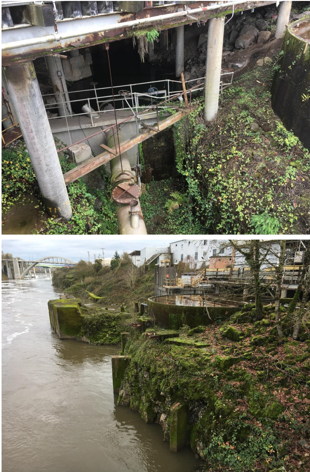
Figure A-3. Photographic views of basalt outcrops and rock debris located near the millrace outlet beneath No. 3 Paper Machine Building #2 (top) and the Circular Tank Foundation 1 (bottom).
