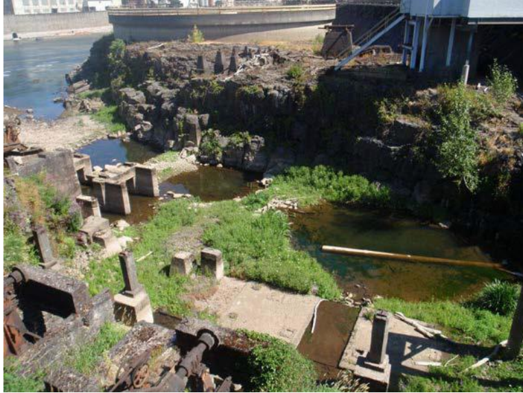
Figure 6. Off-channel alcove habitat surrounded by riparian basalt and remnant infrastructure.
