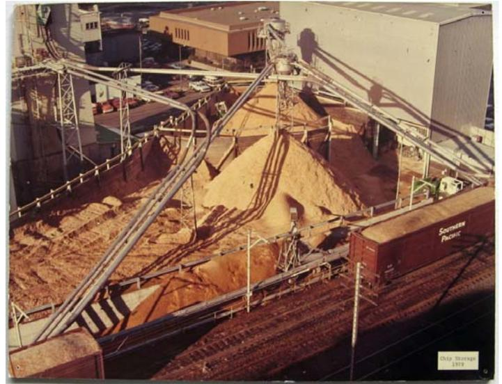
Here you can see a pile of wood chips in 1979 on their way to being cooked and ground into pulp at the paper mill.
